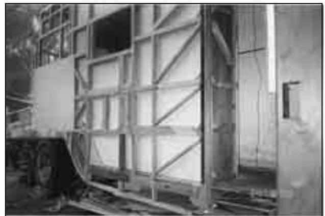
*This was the view of the near side prior to cladding. Note how the interior of the kitchen had to be finished before the cladding went on.*
